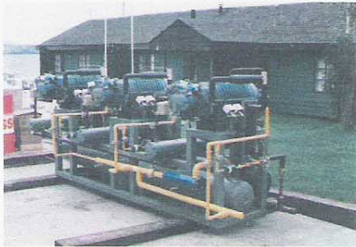
Rack motocompresores
